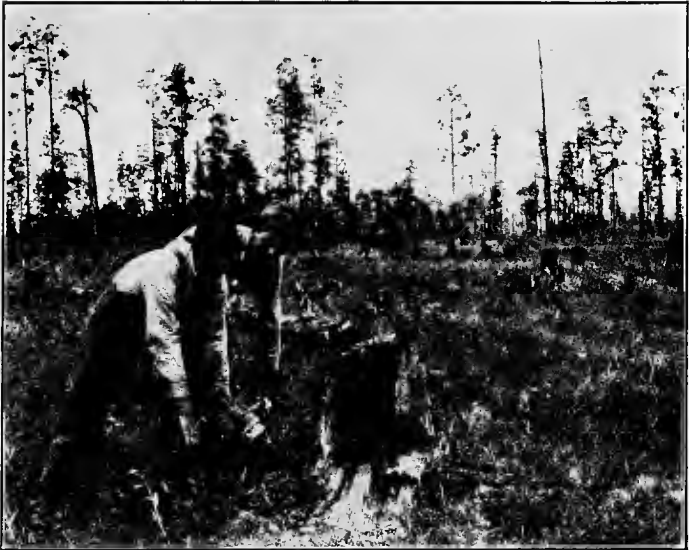
Fig. 24. Boring a Long-Leaf Pine Stump with an Electric Drill
